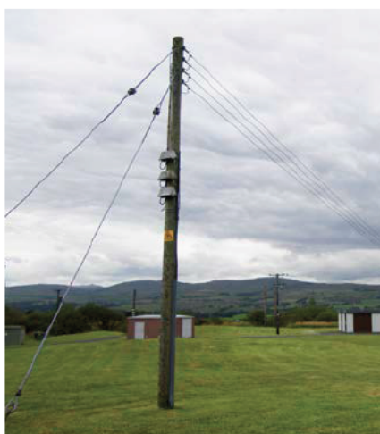
Figure 3 400 V distribution line
