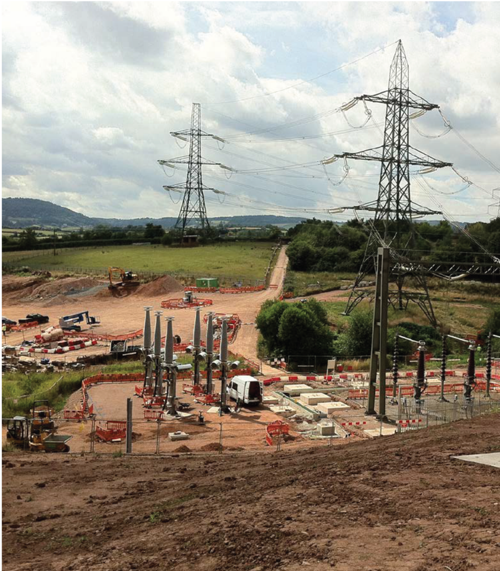
The undergrounding of electricity cables at Ross-on-Wye
